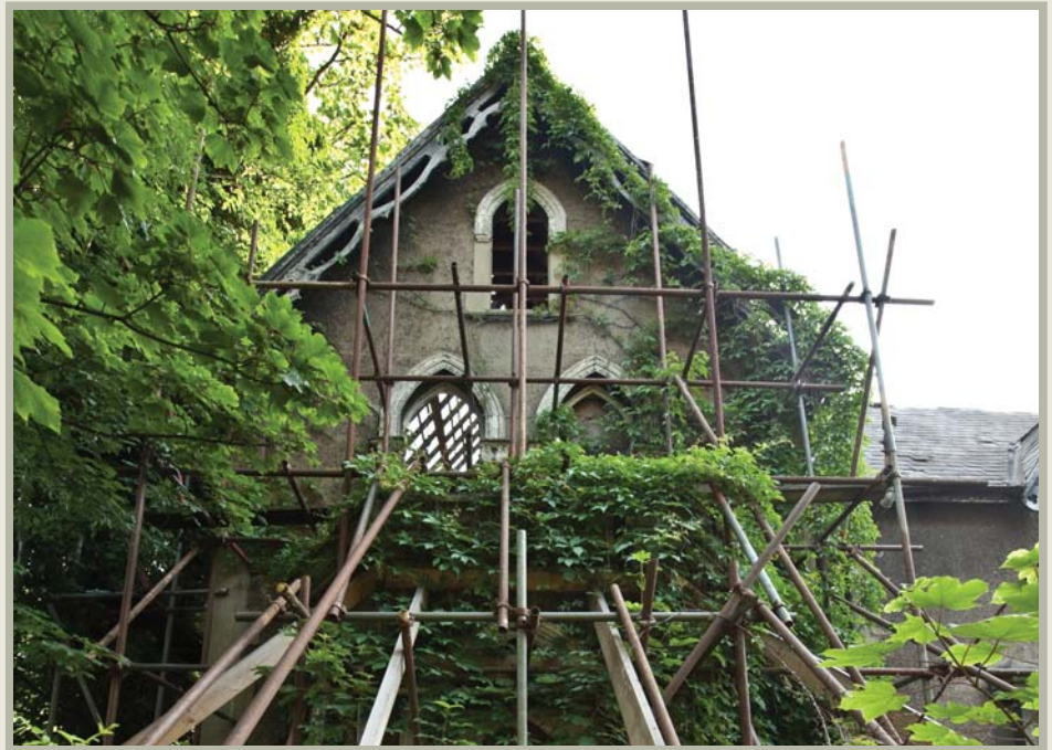
Image Lordship Lane, Southwark. Grade II listed house of 1873. Empty and neglected for many years and suffering from serious structural problems. Local authority is taking action against the owner.
