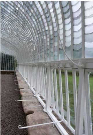
The glasshouse at Felton Park was erected around 1830 to designs attributed to John Claudius Loudon. It measures 90 x 30 feet and stands against an 18th-century brick garden wall that is over 13 feet high. The slender, curved roof, of wrought iron glazing bars with delicate panes of fish-scale glass, rests elegantly
