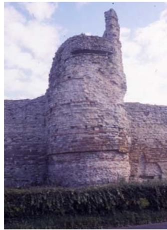
Fig 8. Bastion of the Saxon Shore fort of Pevensey. The upper part of the tower is a concealed Second World War pillbox. Note the slit for a machine gun.
