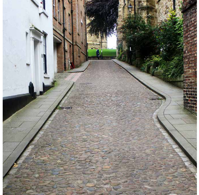
Bow Lane, Durham. This carefully re-laid cobbled surface provides a beautiful and durable lane in the historic heart of the city. As here, smooth paving should also be provided at crossings to assist users of wheelchairs or buggies. © Durham County
